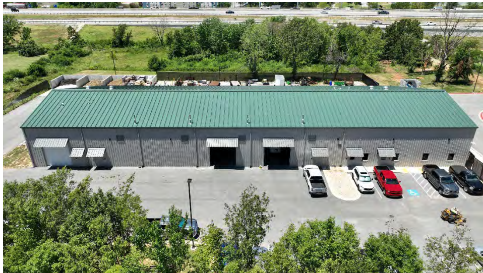
Figure 12. Overview of physical plant building (10).
