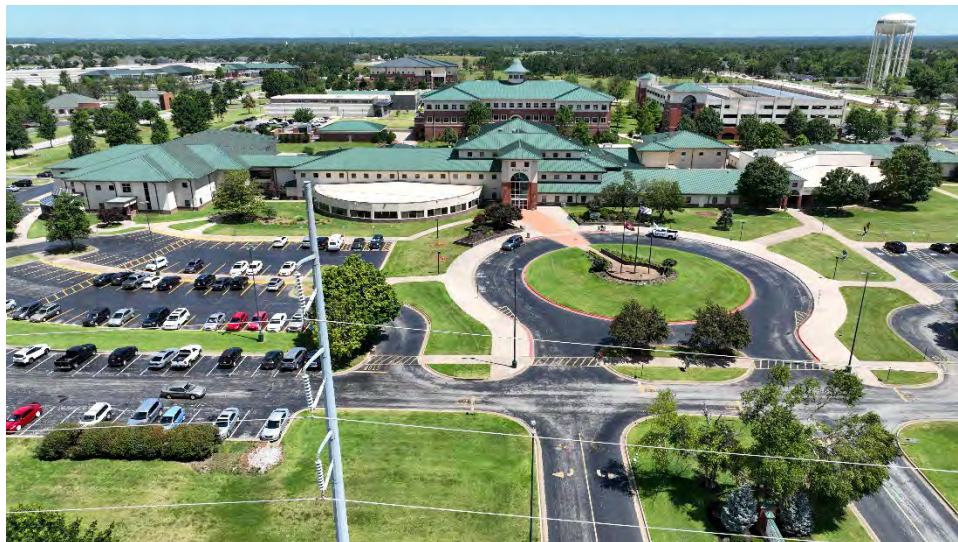
Figure 3. Overview of Bob Burns hall (1).
