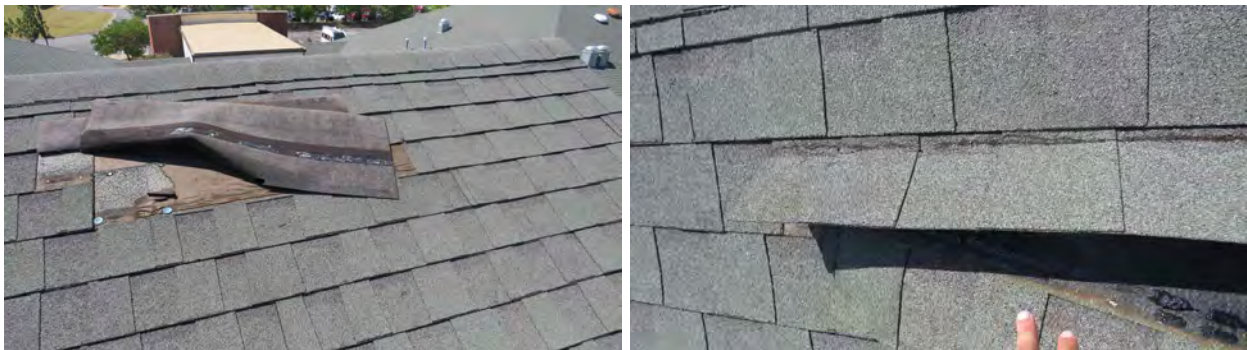
Figure 96. Roofing on the national child protection training center (8) with wind-related conditions.
