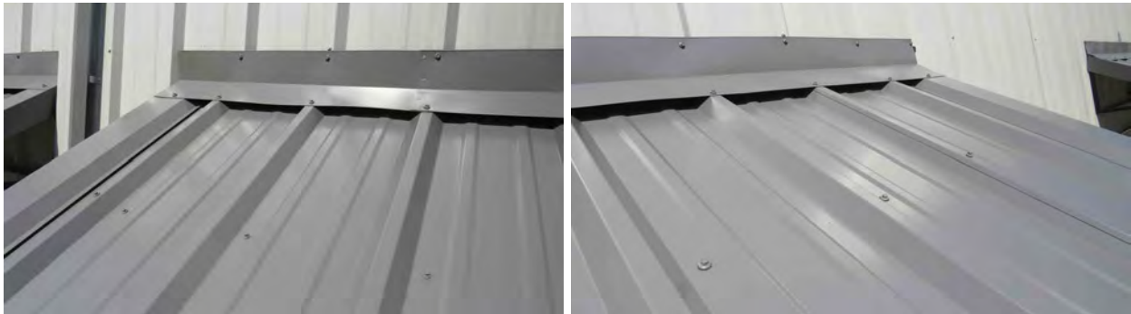
Figure 66. Roofing on the physical plant building (10) with no wind damage.
