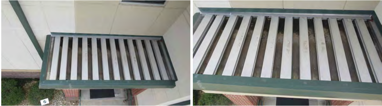
Figure 65. Roofing on the bob burns hall (1) with no wind damage.
