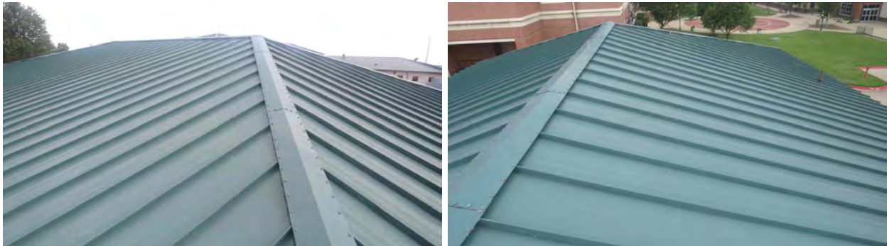
Figure 75. Roofing on the central energy plant (3) with no wind damage.
