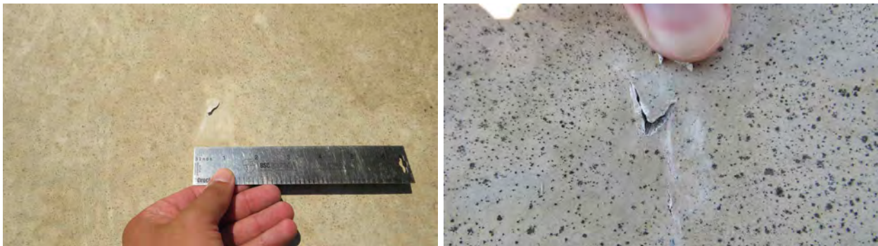
Figure 90. Roofing on the bob burns hall (1) with wind-related conditions.
