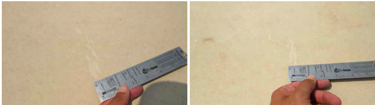
Figure 48. Roofing on the integrated design lab (6) with no hail damage.
