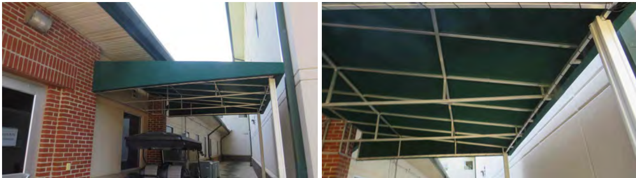
Figure 98. Roofing on the Bob Burns hall (1) with no wind damage.
