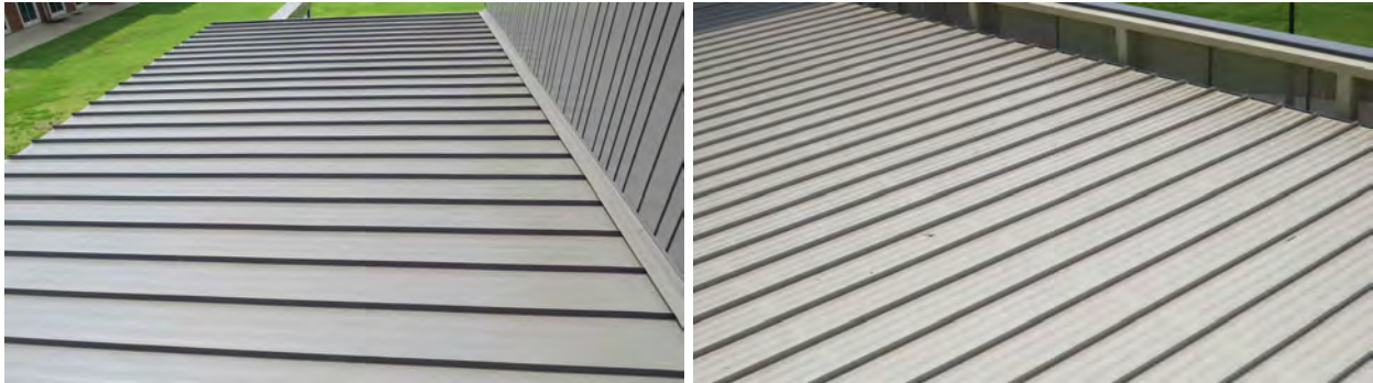
Figure 74. Roofing on the integrated design lab (6) with no wind damage.
