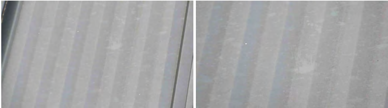
Figure 18. Roofing on the center for health professionals (2) with no hail damage.
