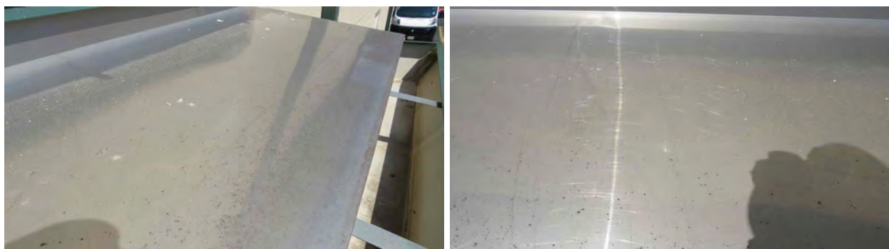
Figure 45. Roofing on the bob burns hall (1) with no hail damage.
