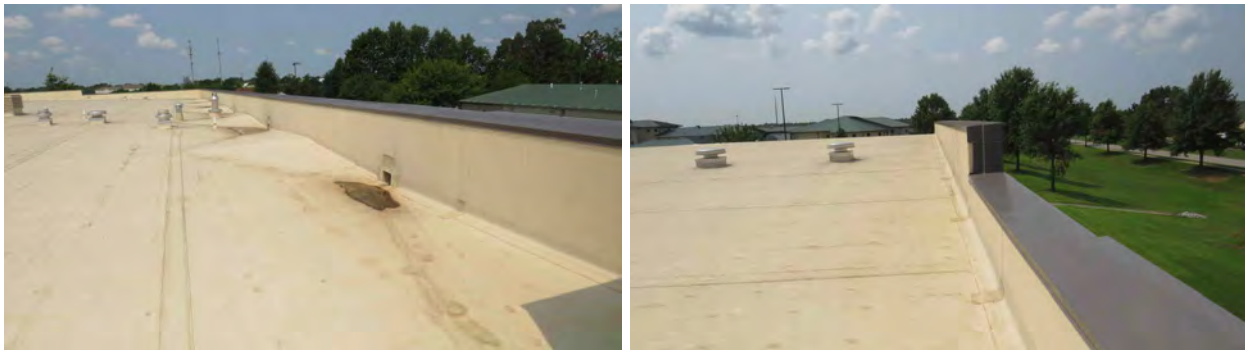
Figure 88. Roofing on the integrated design lab (6) with no wind damage.
