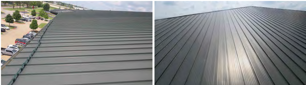
Figure 76. Roofing on the center for health professionals (2) with no wind damage.
