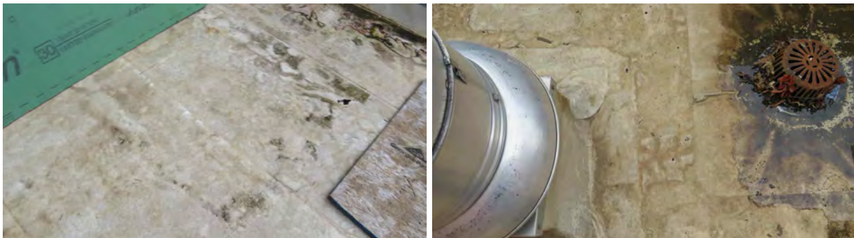
Figure 41. Roofing on the student center (13) with no hail damage.
