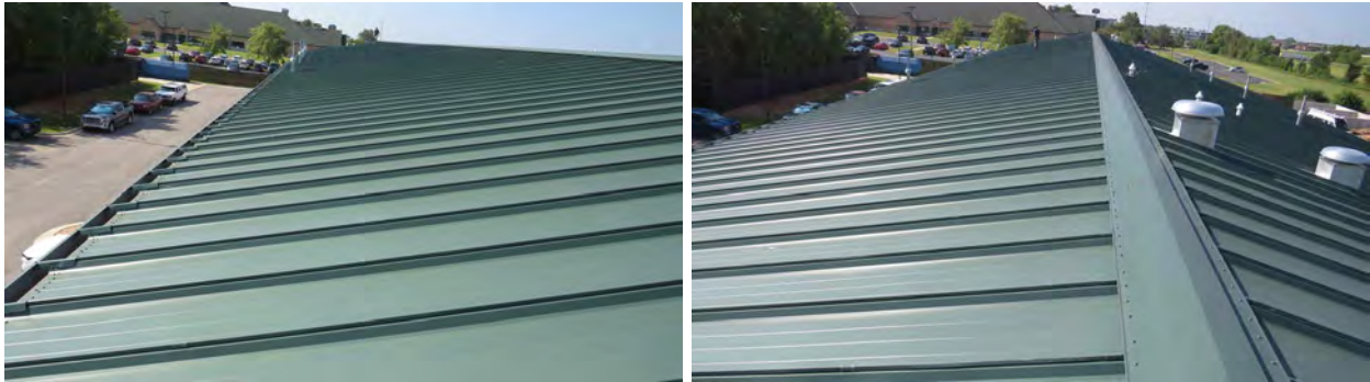
Figure 85. Roofing on the physical plant building (10) with no wind damage.
