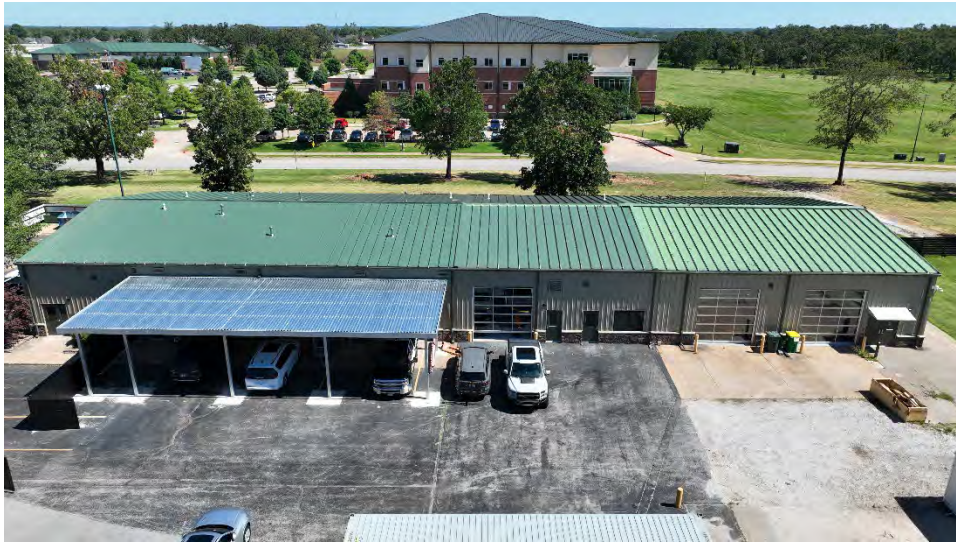
Figure 9. Overview of maintenance building (7).
