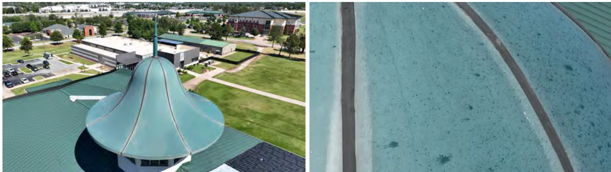
Figure 46. Roofing on the student center (13) with no hail damage.
