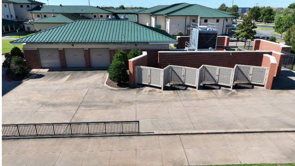
Figure 5. Overview of central energy plant (3).
