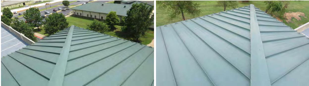
Figure 78. Roofing on the parking structure (9) with no wind damage.
