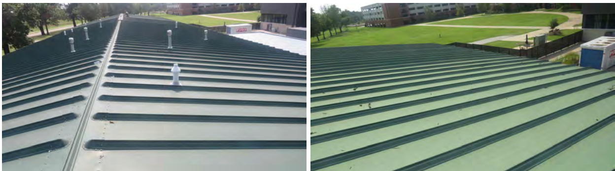
Figure 87. Roofing on the maintenance building (7) with no wind damage.
