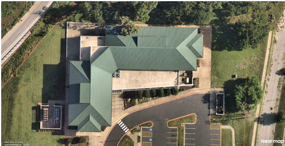
Figure 55. Nearmap image of the shrewmaker center for workforce tach (12) captured on May 27, 2024.
