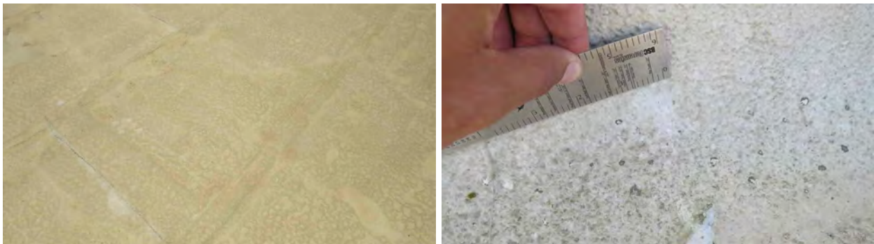
Figure 38. Roofing on the national child protection training center (8) with no hail damage.
