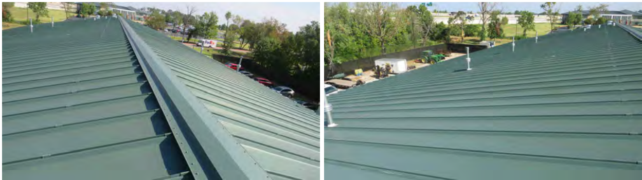
Figure 84. Roofing on the physical plant building (10) with no wind damage.
