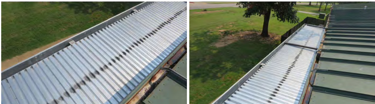
Figure 68. Roofing on the maintenance building (7) with no wind damage.
