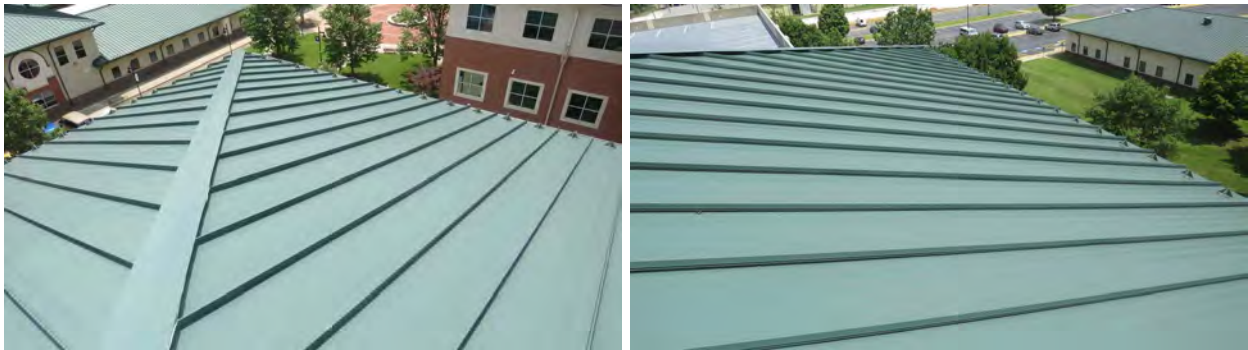
Figure 77. Roofing on the parking structure (9) with no wind damage.
