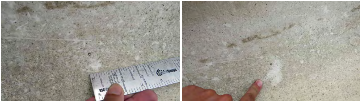
Figure 39. Roofing on the global business development center (5) with no hail damage.
