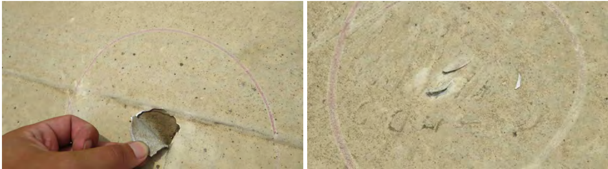
Figure 93. Roofing on the global business development center (5) with wind-related conditions.
