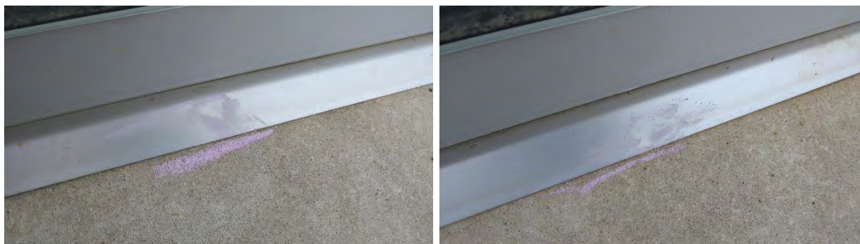
Figure 2. Vulnerable elements with evidence of historical hailfall.
