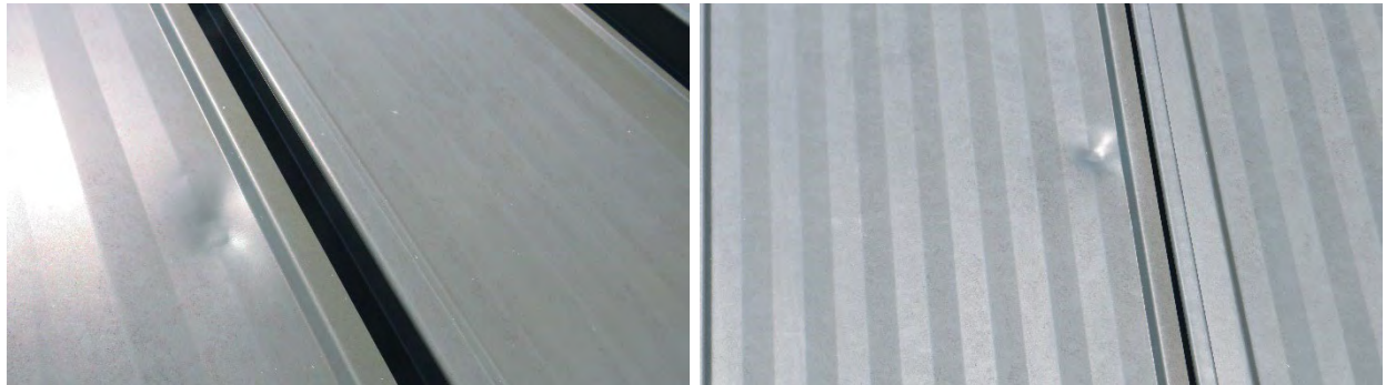
Figure 79. Roofing on the shrewmaker center for workforce tech (12) with wind-related conditions.
