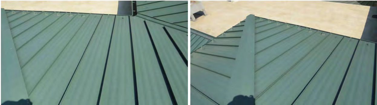
Figure 70. Roofing on the bob burns hall (1) with no wind damage.
