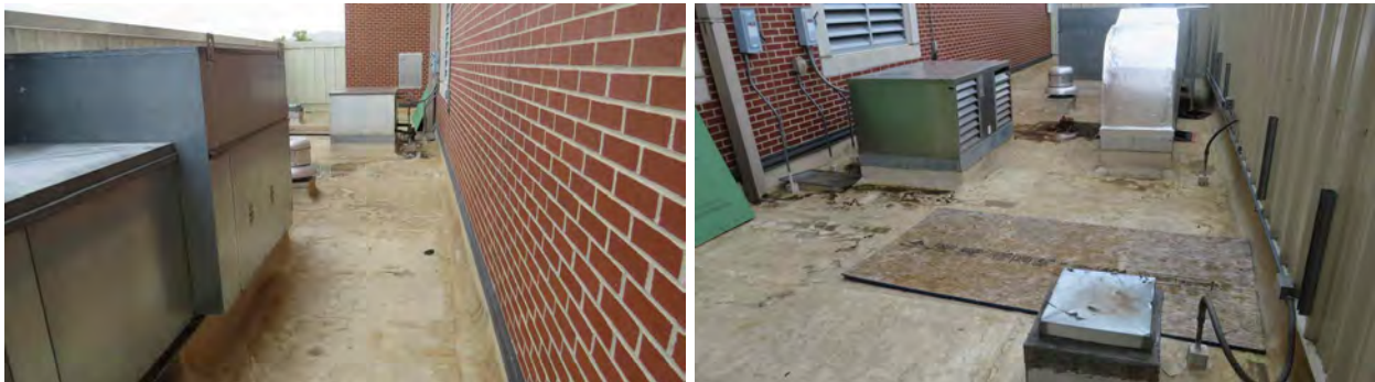
Figure 94. Roofing on the student center (13) with no wind damage.
