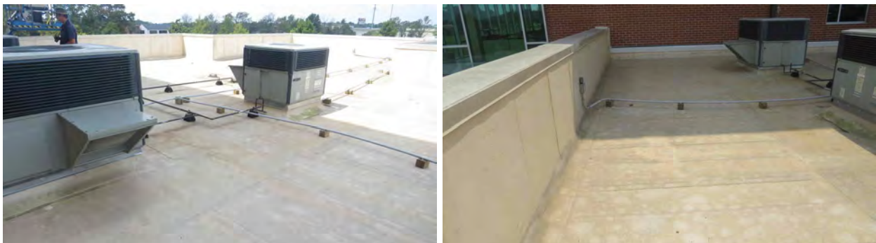
Figure 95. Roofing on the center for health professionals (2) with no wind damage.
