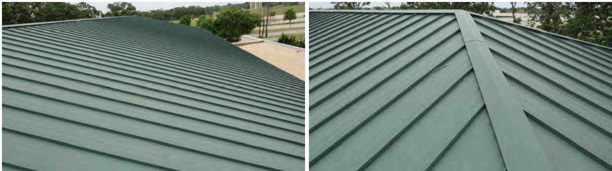
Figure 73. Roofing on the global business development center (5) with no wind damage.
