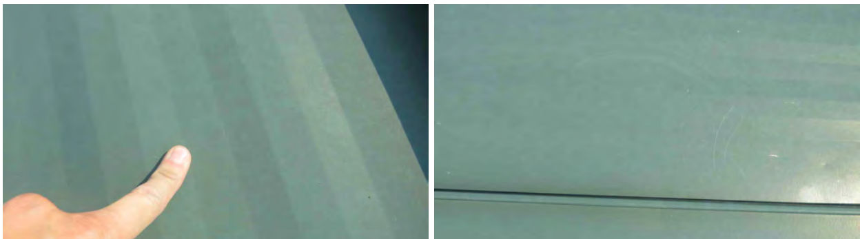
Figure 20. Roofing on the student center (13) with no hail damage.
