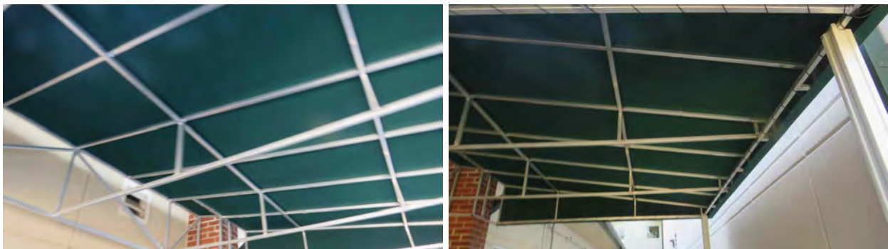
Figure 52. Roofing on the Bob Burns hall (1) with no hail damage.
