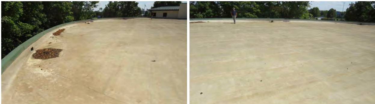
Figure 91. Roofing on the bob burns hall (1) with no wind damage.
