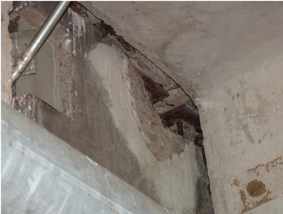
Photo 2. Typical concrete beam spalling.
