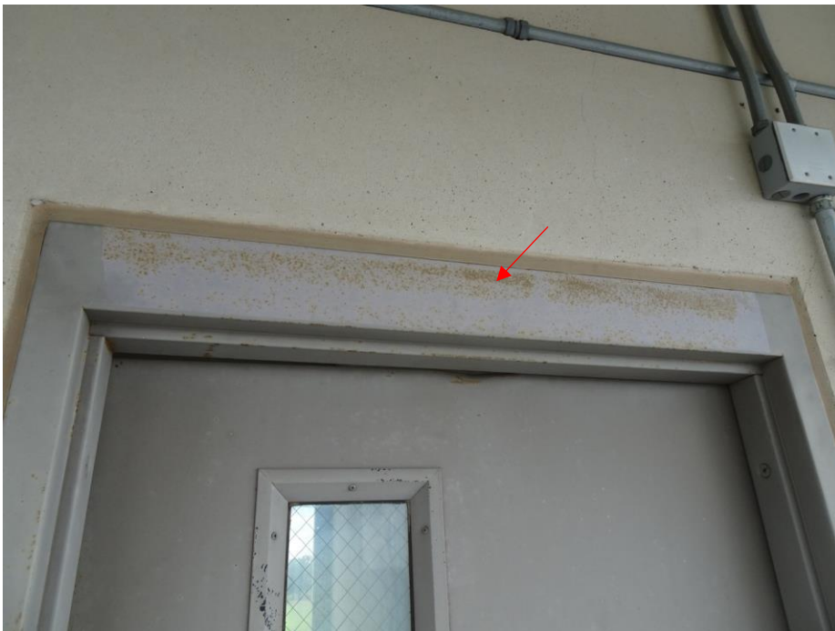
Photo 22. Corroded door frame on Level 5.
