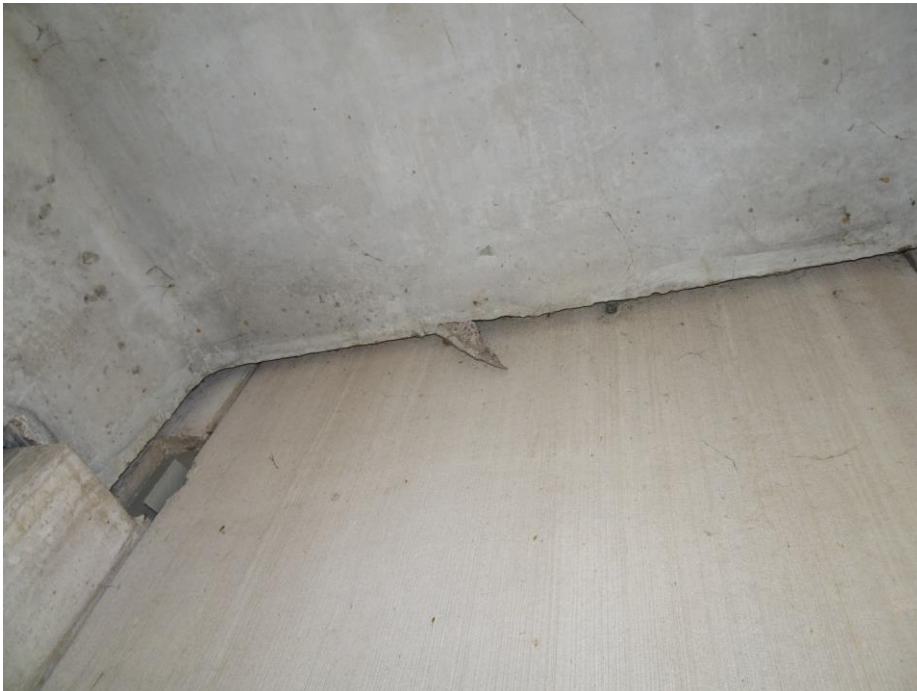
Photo 12. Loose overhead concrete indicative of a falling debris hazard at Level 1.
