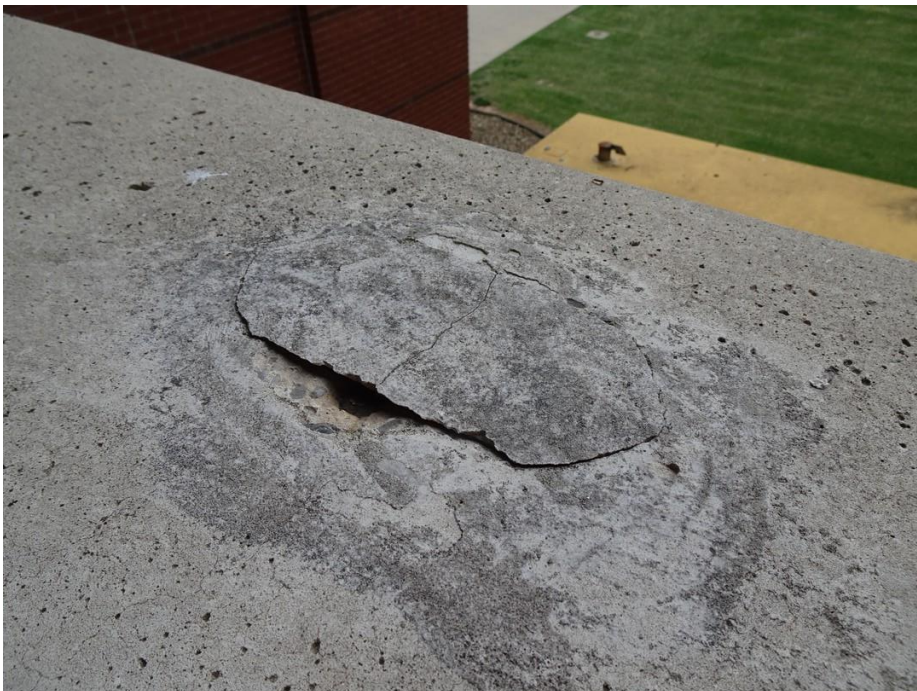
Photo 14. Close-up view of deteriorated grout pocket located on Level 2.
