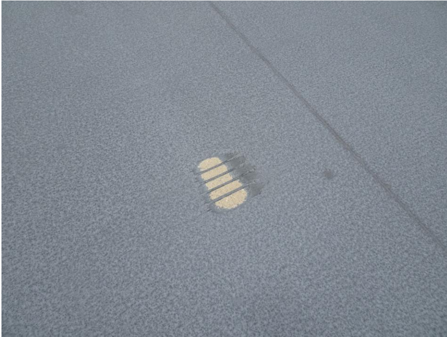
Photo 20. Faded traffic markings on the fifth level.
