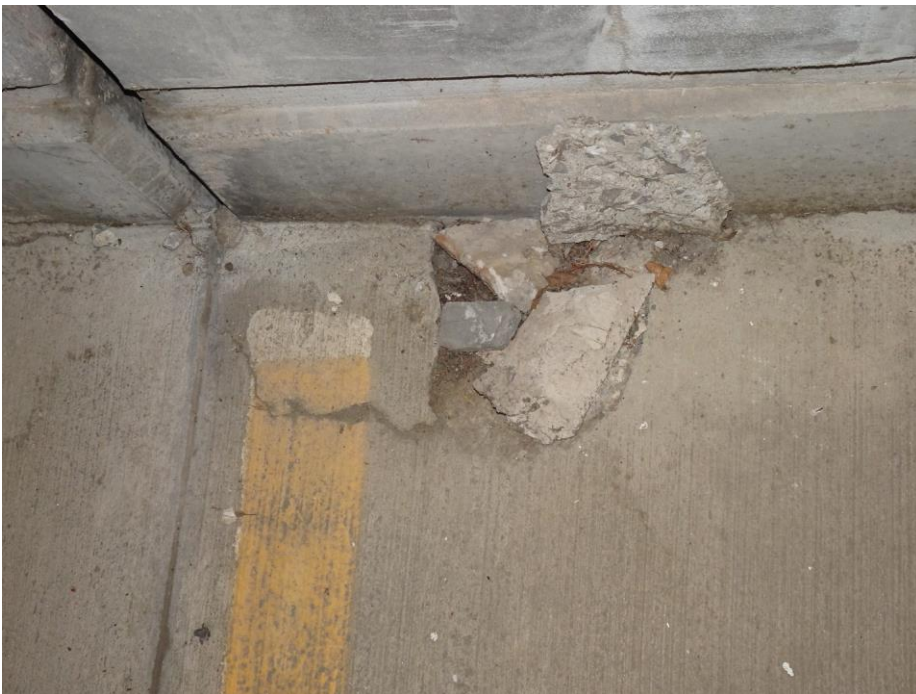
Photo 10. Close-up view of typical concrete floor spalling.
