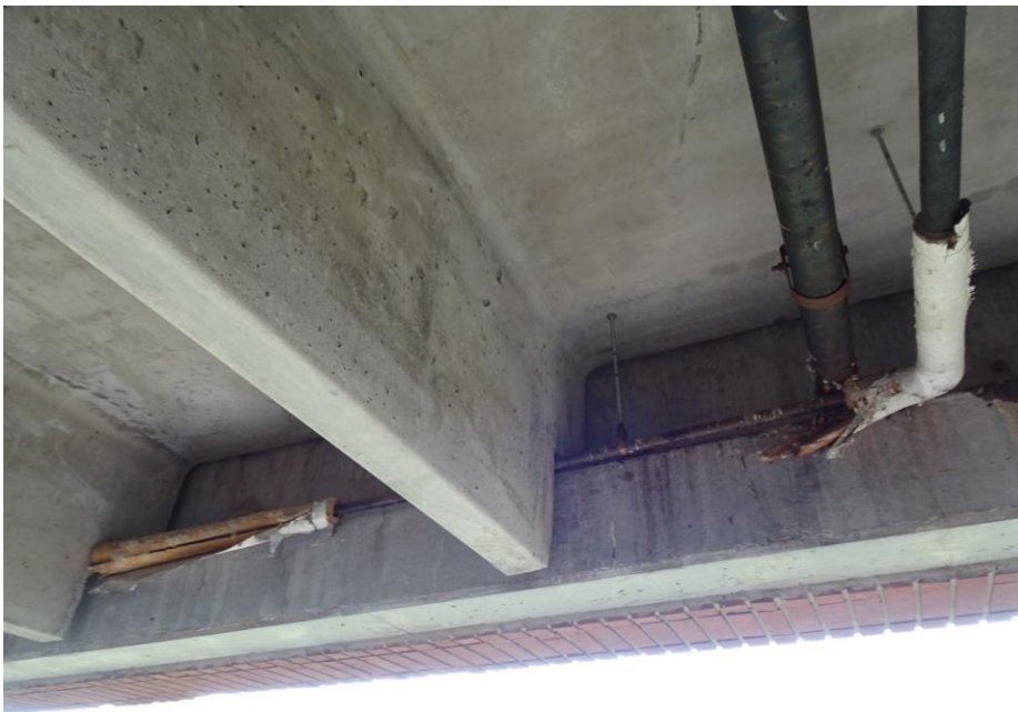
Photo 26. Damaged piping at Level 1.
