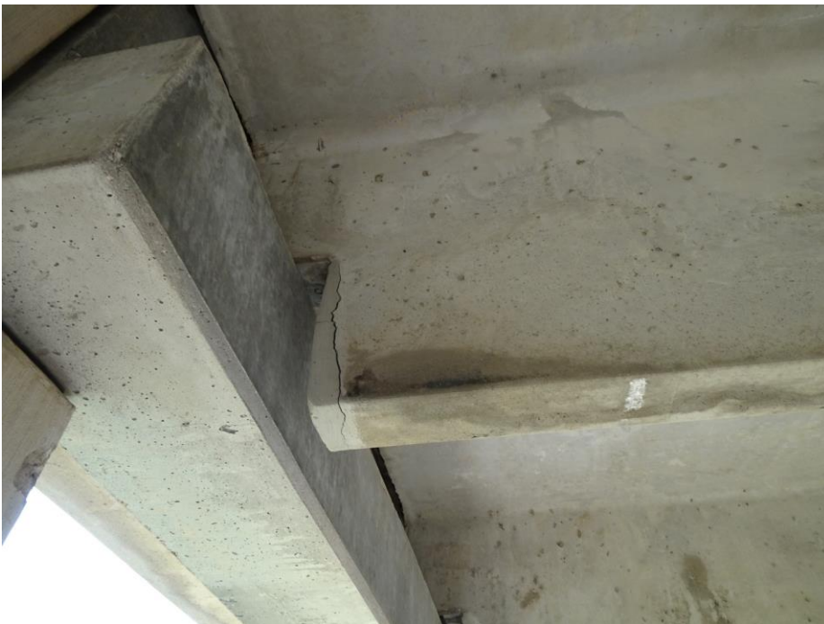
Photo 4. Concrete double-tee stem spalling.
