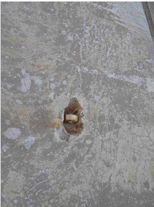
Photo 16. Close-up view of typical ungrouted anchors.
