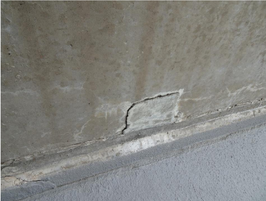
Photo 16. Close-up view of typical ungrouted anchors.
