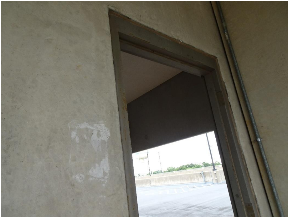
Photo 28. Missing level sign on level 5.
