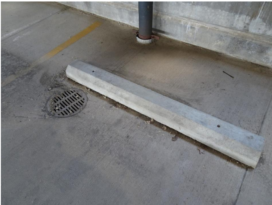
Photo 24. Typical wheel stops not painted yellow.
