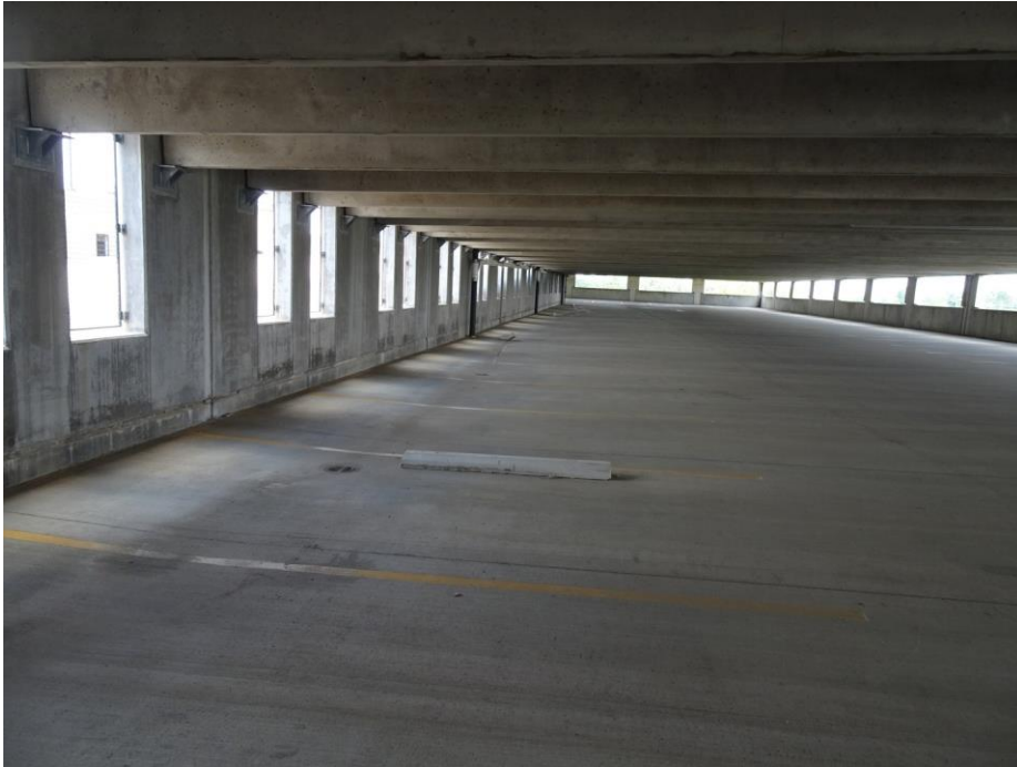
Photo 24. Typical wheel stops not painted yellow.
