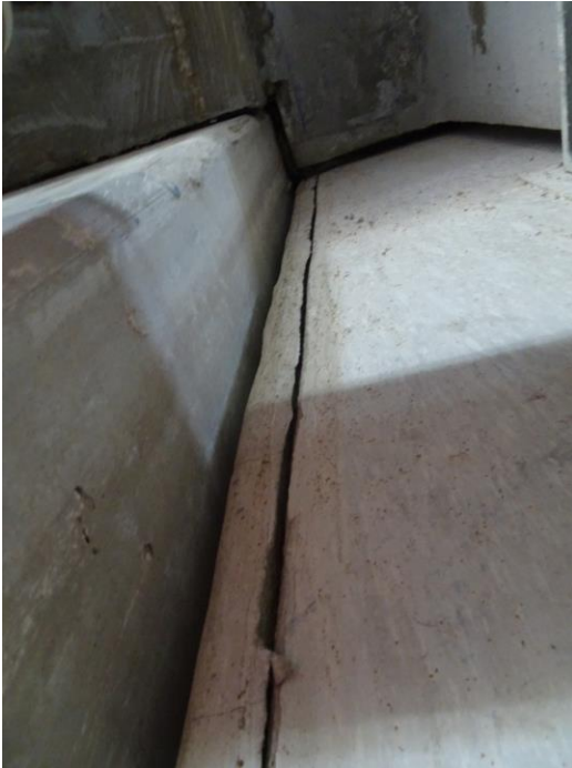
Photo 10. Close-up view of typical concrete floor spalling.
