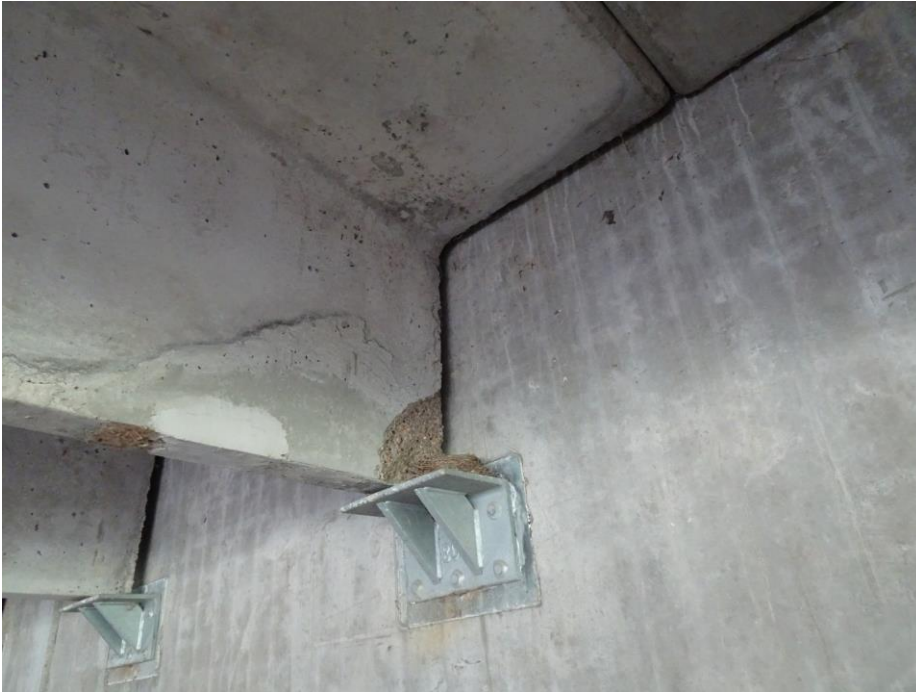
Photo 4. Concrete double-tee stem spalling.
