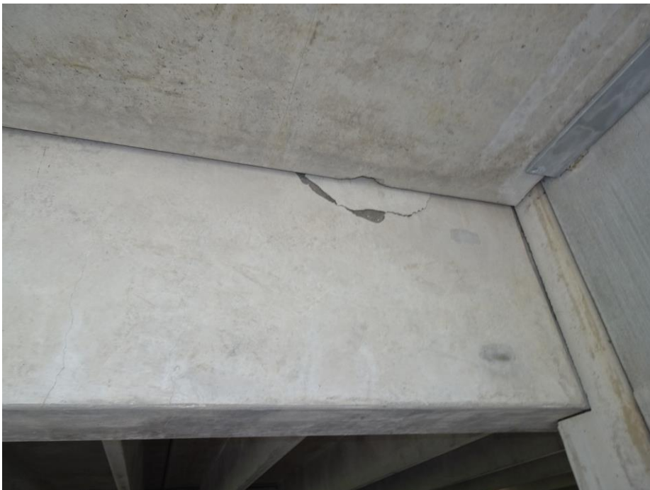
Photo 2. Typical concrete beam spalling.
