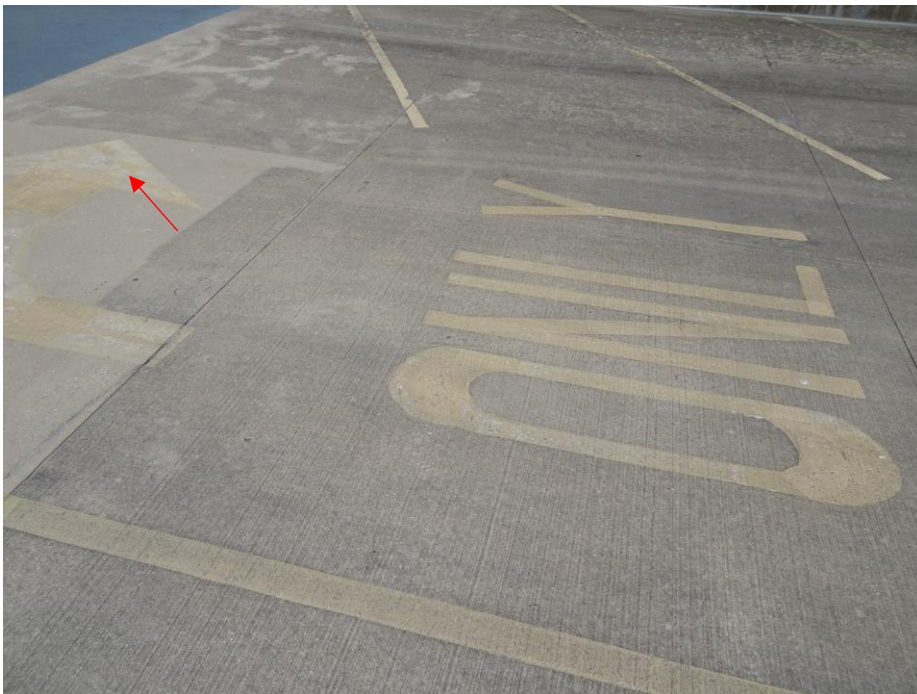
Photo 20. Faded traffic markings on the fifth level.
